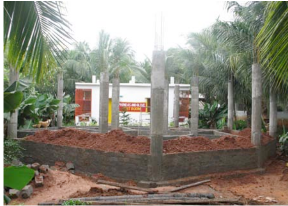
Ongoing construction for octagon house for the dogs
